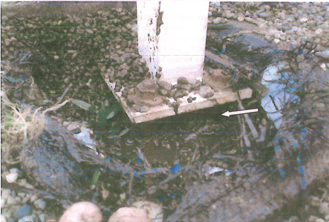
11 – The aluminium rails which surround several of the areas on the main roof were installed directly into the roofing membrane. The bolts which support it have suffered extensive corrosion
