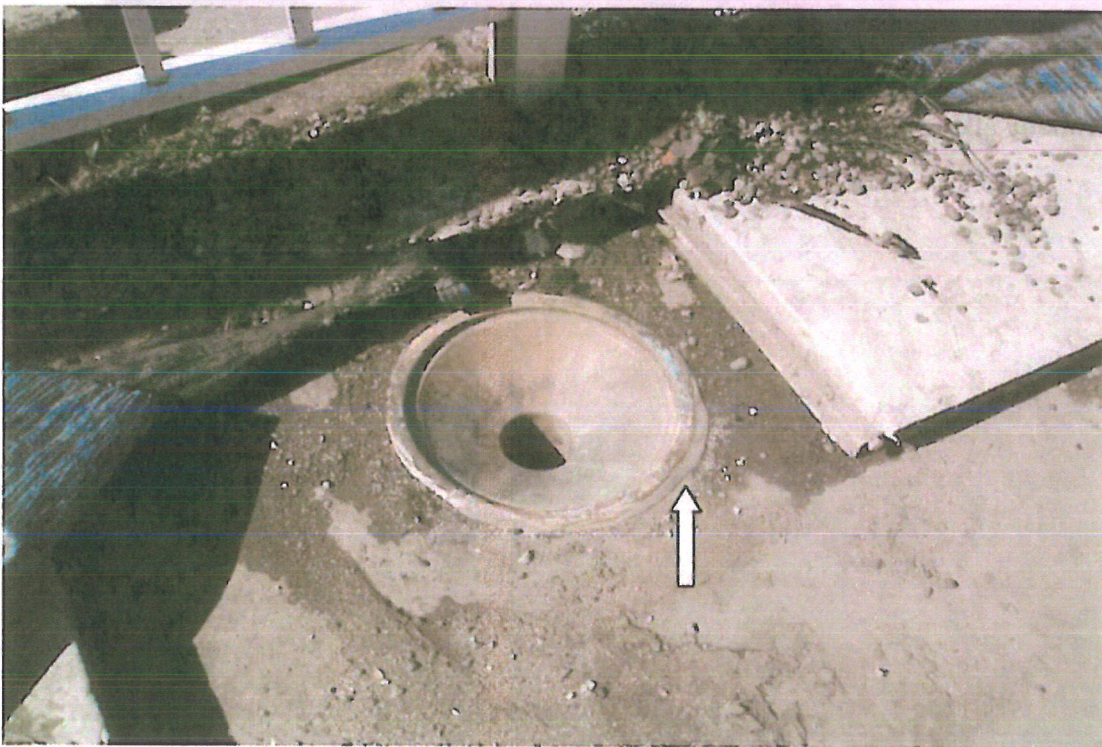
17 – The drain shown in this photo is part of the area which was cleared off in order to locate the source of water ingress. The drain screen was removed and could potentially allow debris to
