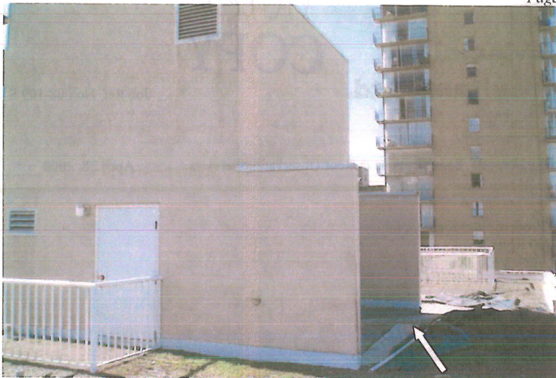
1 – This overview shows the main roof area as well as the upper elevator shaft roof. Notice the large area where the insulation and ballast has been removed in an attempt to locate the source of ingress in # 802. Also notice the paving stones and the metal railings which have been incorporated into the roof assembly.
