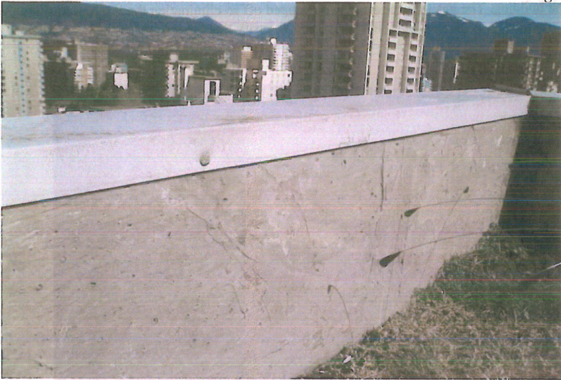
10 – The rubber membrane on some of the walls is very thin which has resulted in exposed concrete. Again these areas have potential to allow water to ingress the building.
