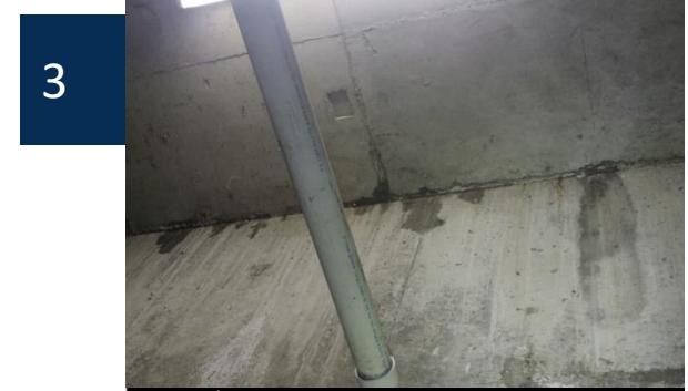
Water ingress at wall and ceiling transition, from level above.
