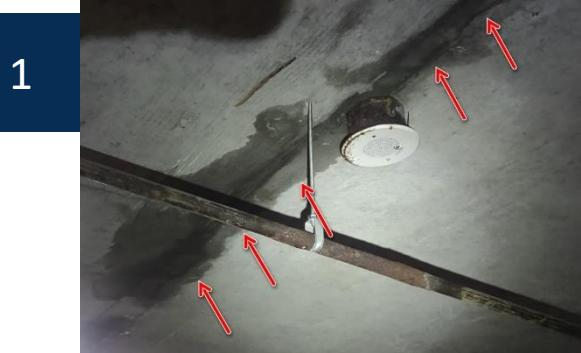
Active water ingress originating from Level 1, and rusted speaker.
