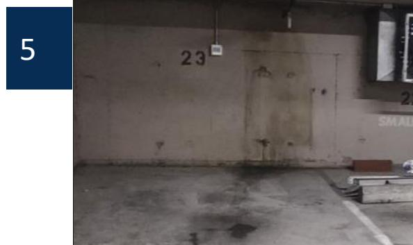
Water infiltrating through planters, slab into the 3<sup>rd</sup> level below.
