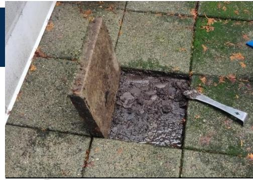
Membrane under patio pavers observed to be in poor condition.
