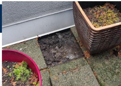
Membrane under pavers observed to have failures throughout.
