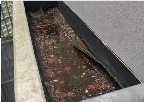
Membrane in unit planter insufficient installation and deterioration.
