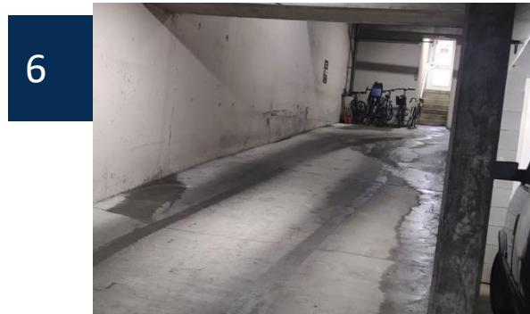
Water infiltrating parkade slab due to insufficient coating and trickling down ramps to other levels.
