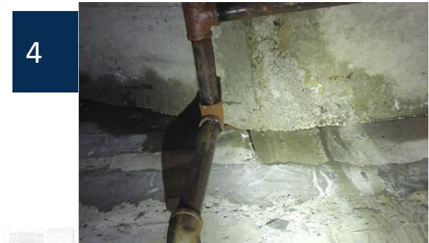
Water infiltrating through exterior foundation walls.
